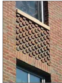
SAMPLE IMAGE PROJECTING BRICK DETAIL PANELS
