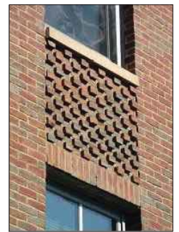
SAMPLE IMAGE PROJECTING BRICK DETAIL PANELS
